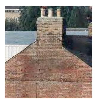
Condensing gases within a flue and terminal can have a corrosive effect on certain materials.
